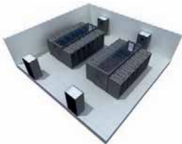
Raised floor data center with perimeter precision cooling (Liebert HPM)
